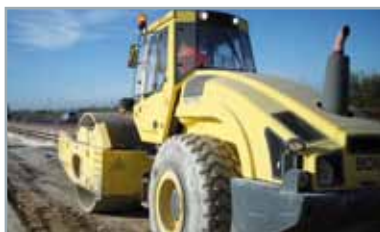
5. Compression of machined and improved road
