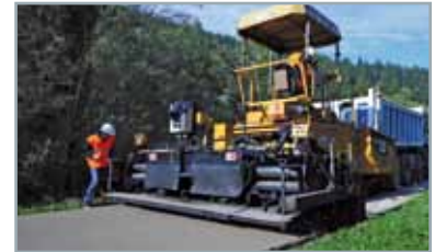
3. Laying of mixture with road finisher
