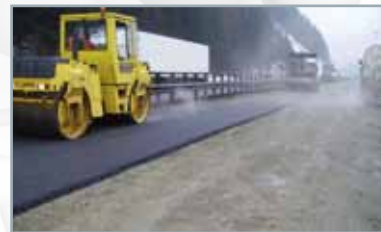
6. If necessary application of asphalt
