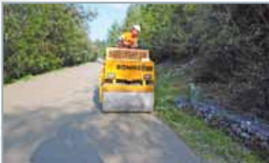
4. Compression and rolling of laid mixture
