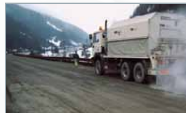
3. Application of binding agent through binding agent spreader
