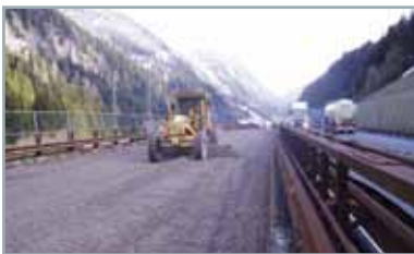
2. Creation and levelling of plane
