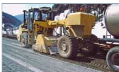
4. Stabilization of on-site existing earth with mixture of Nanoalps® System SOIL
