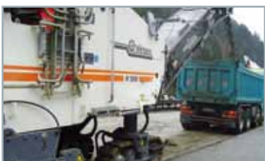
1. Removal of asphalt layer with asphalt milling machine
