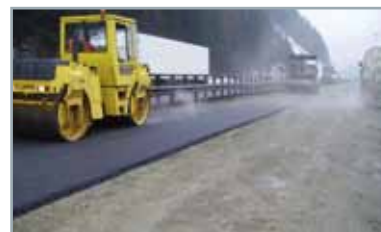
6. If necessary application of asphalt
